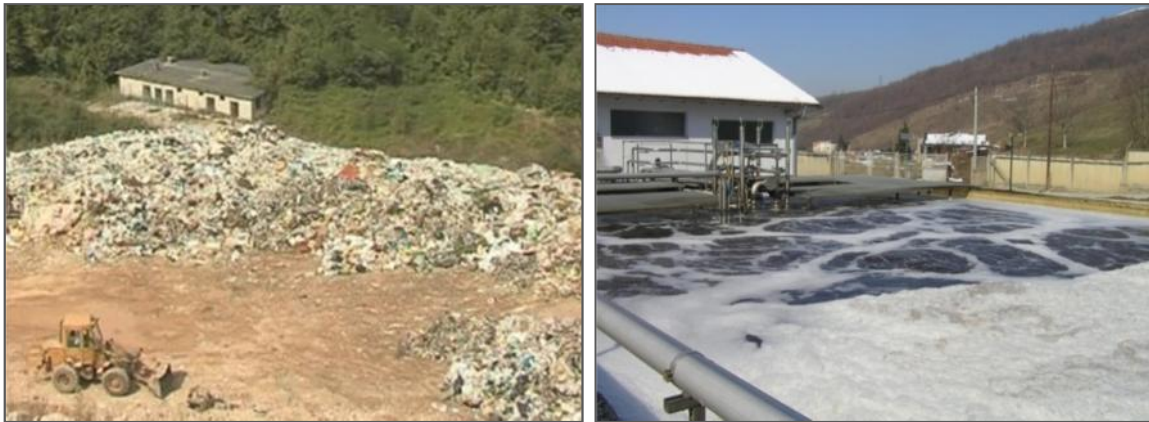
Chaos versus Control: Krupac dumpsite (left) and Canton Sarajevo sanitary landfill (right).
